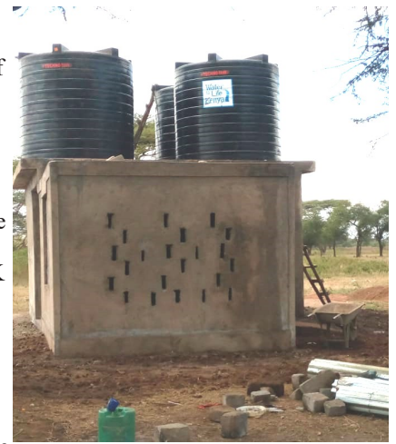
Storage containers are elevated to discourage elephants from knocking them over to access the water.
