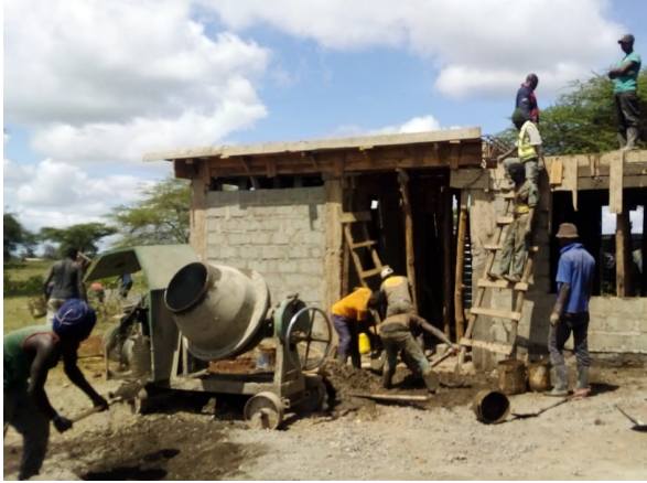
Building a protective house for the diesel generator.
