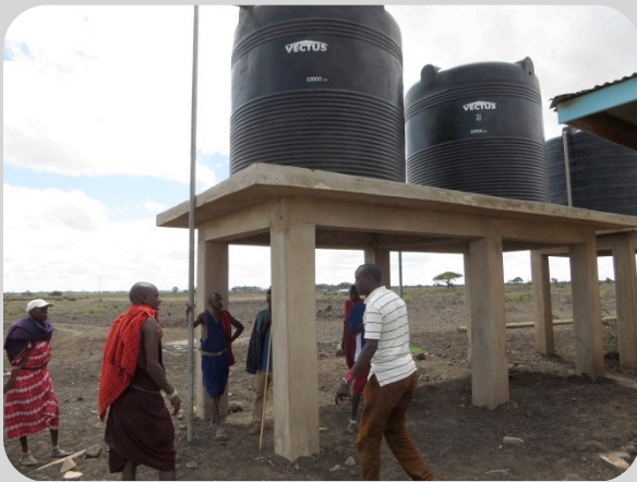
The water tanks at Enkong'u Narok
